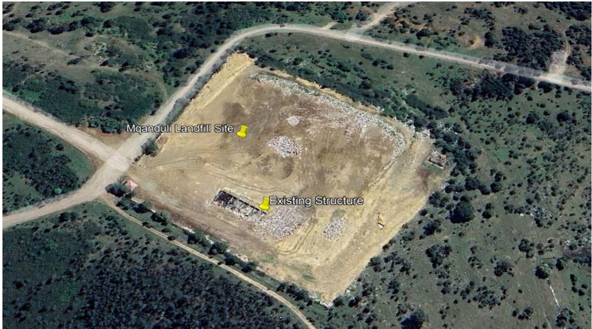
Figure 1: indicates the Mqanduli Landfill Site
