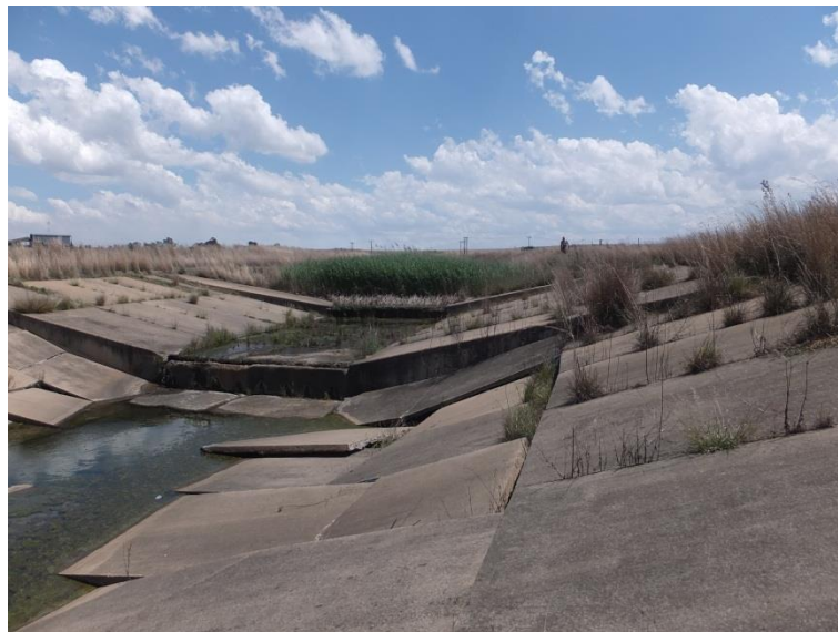
Figure 3. Novel passive treatment system installed at a coal mine discharge point in Mpumalanga. This device aims to agitate a lime-AMD slurry using a vertical-axis wind turbine. At the time that this photograph was taken, the system was not functioning due to the breakage of the turbine.
