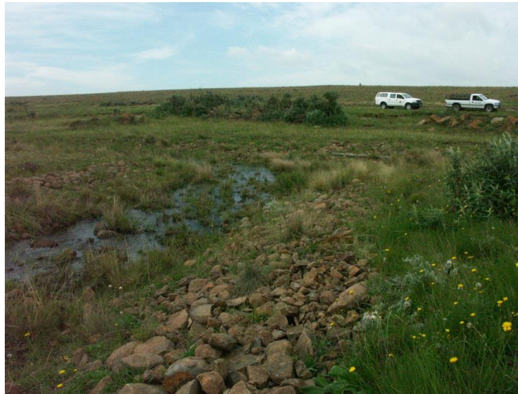
Figure 5. Ingress prevention by the sealing of channels above underground coal workings - Kwazulu Natal
