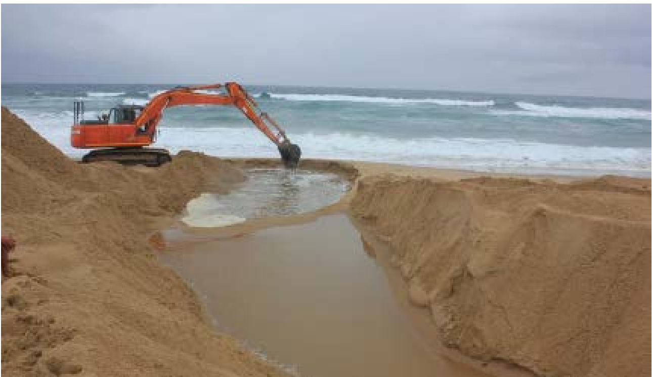
Artificially breaching the mouth of an estuary is a complex process that must be carried out following a mouth-breaching protocol that has been developed for the particular estuary. Unnecessary and inappropriate breaching can have significant negative impacts on the ecological functioning, including loss of blue carbon ecosystems. Here the St Lucia Estuary (KwaZulu-Natal) is breached (Photo: C Fox).
