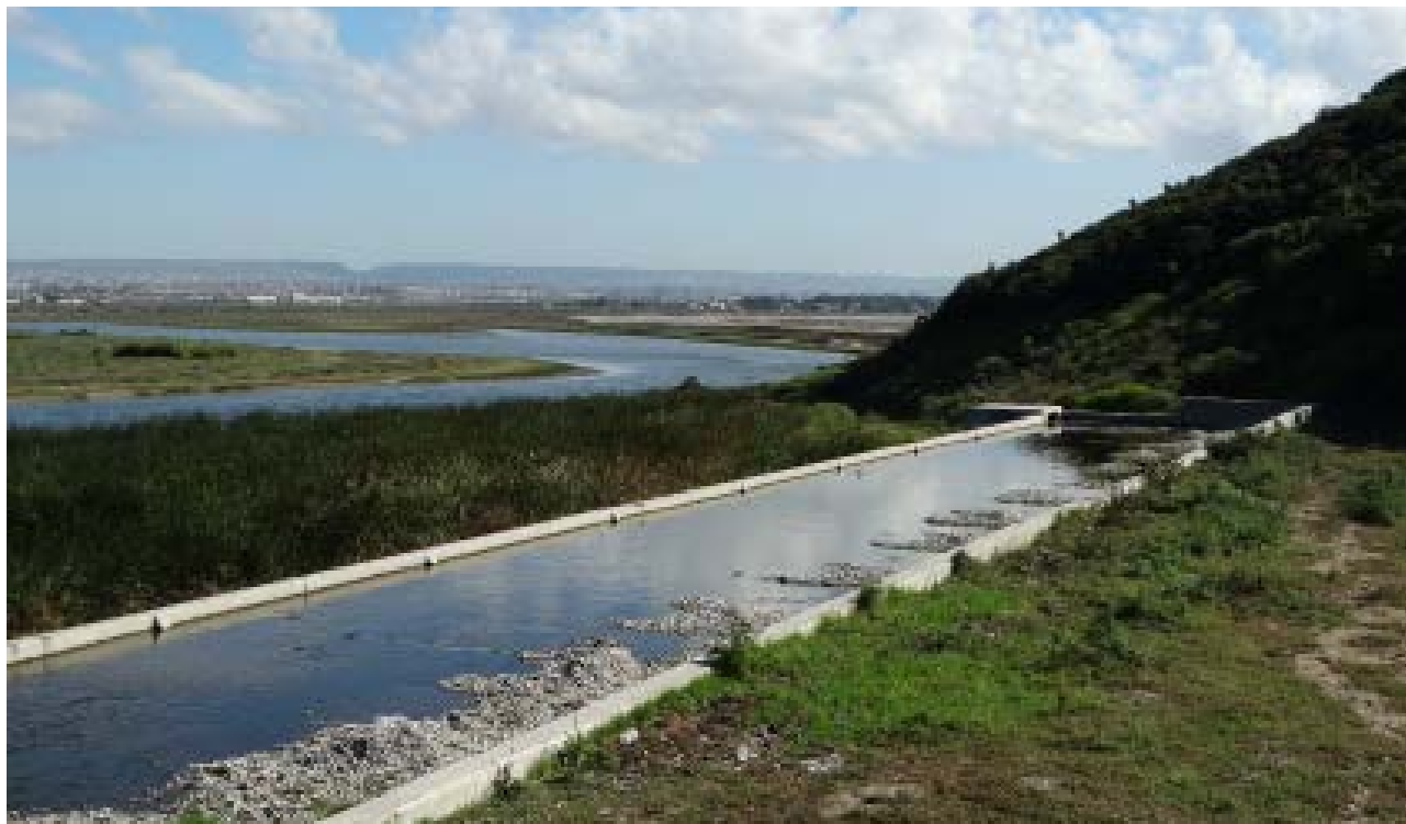
Reduced water quality and eutrophication in blue carbon ecosystems occurs when effluents from WWTWs, urban stormwater or agricultural runoffs flow into the estuarine environment. Artificial wetlands present a sustainable development approach to filter such inputs. Shown here is one at the Swartkops Estuary which drains runoff from the Motherwell area (Gqeberha, Eastern Cape) (Photo: J Adams).
