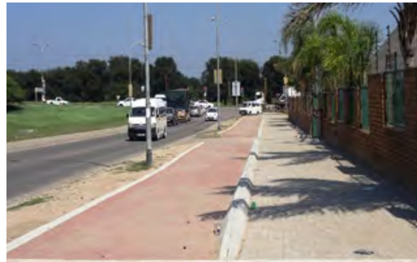
Figure 5.7 Polokwane Pilot Project – Separation of Bicycling and Pedestrian routes
