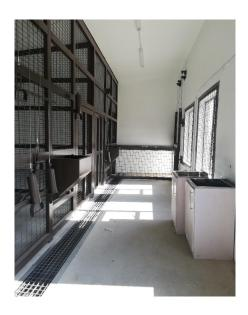
Example of the animal keeper's area within a lion house. Welded mesh over the windows, drains in keepers area, feeding bins, easy to clean floors, and a mesh tunnel connecting the house to the feeding area.
