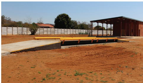
Figure 19 Weighbridge and waste sorting facility at Phokeng Buy back centre in, North West Province
