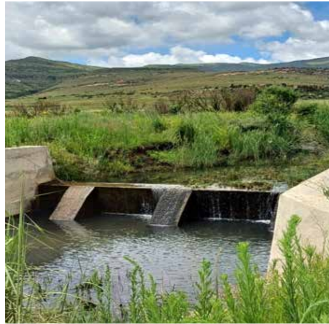
Above: Concrete buttress weir.
