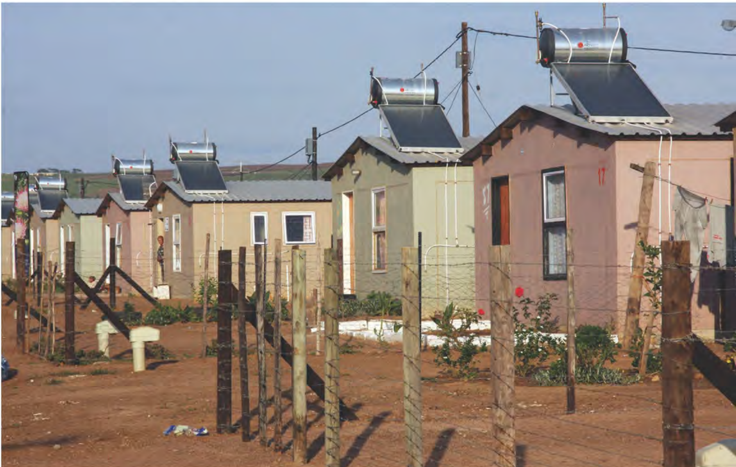
Newly fitted solar water geysers in Darling, Western Cape.
