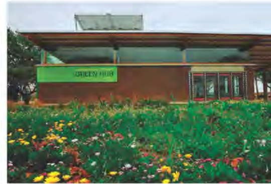
Umgeni River Estuary Green Hub Building (eThekweni Municipality, 2010)
