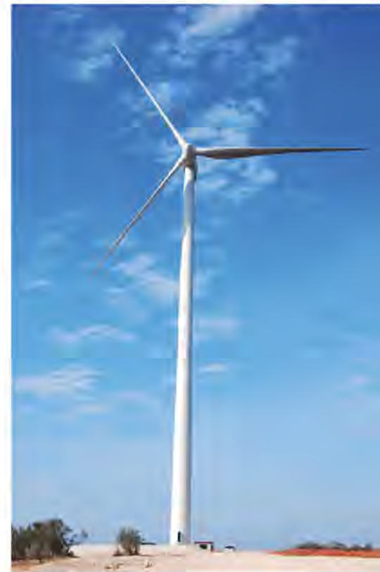
First Electrawinds Wind Turbine at Coega IDZ.
