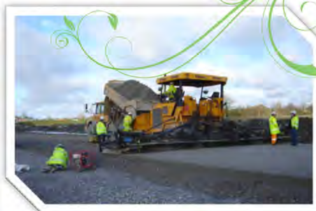
Figure 21: Refuse derived fuel bales ready for gasification; gasification ash residues used as aggregate for road building (image courtesy of Ballast Phoenix)
