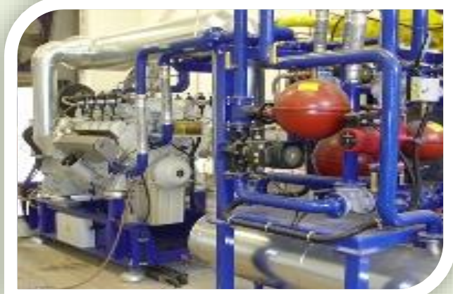
Figure 3-15: Biogas CHP engine and cleaning equipment (image courtesy of WolfeWare Ltd)
