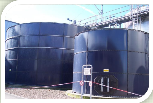
Figure 3-14: Anaerobic digestion tanks (image courtesy of WRAP)
