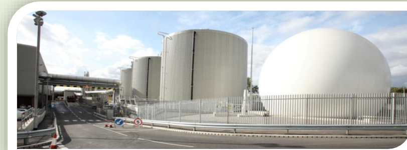
Figure 3-11: Anaerobic digestion and gas storage (Viridor)
