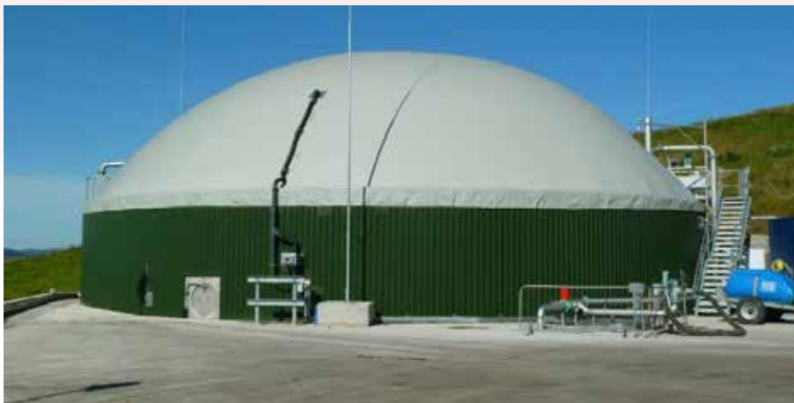
Figure 6.10: Digester with foil roof for gas storage (Anaergia)
