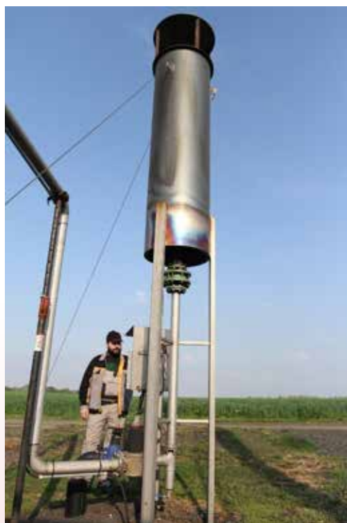
Figure 6.11: Gas flare of a biogas plant (Anaergia)
