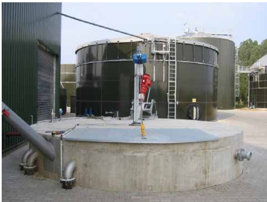
Figure 6.2: Storage for liquid feedstock (Fachverband Biogas e.V.)
