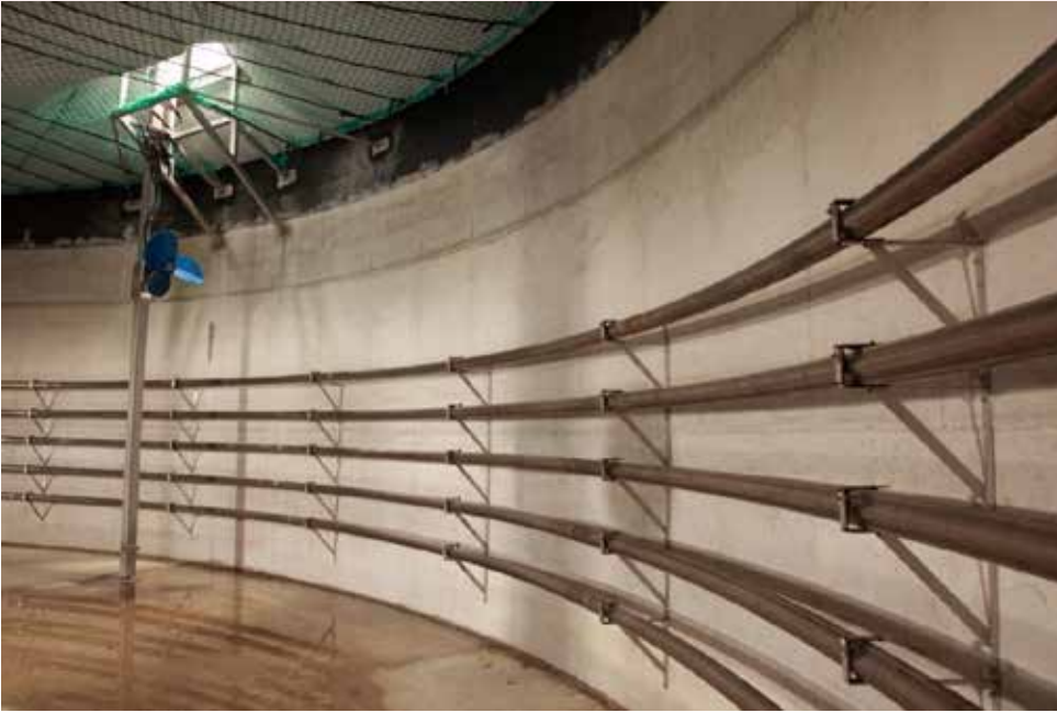
Figure 6.9: Heating system showing pipes containing hot water on the inner digester walls (Anaergia)
