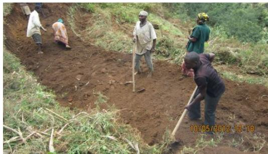
**Figure 7: Excavation of terraces in Tanzania**
