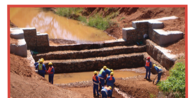
Working for Land beneficiaries building a water pathway.
