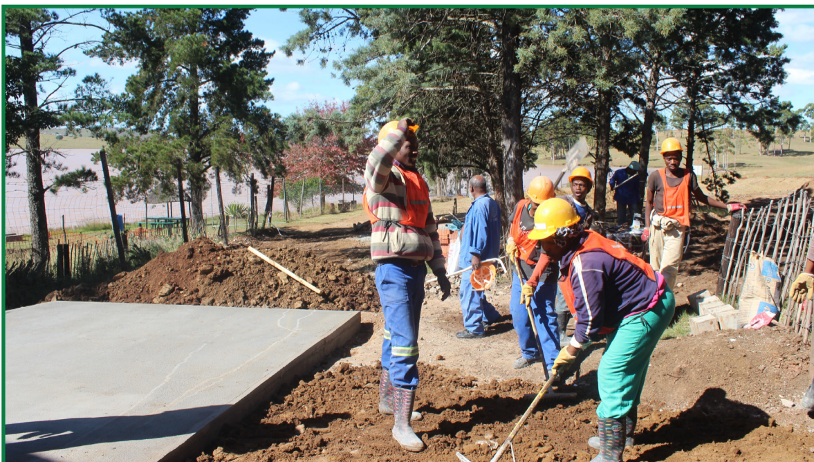
PICKING HER SPOT: Mthatha Dam Tourism and Recreational facility during construction.
