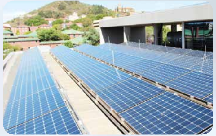
Above: The roof is covered with solar photovoltaic panels to supply almost 20% of the building's energy needs.
