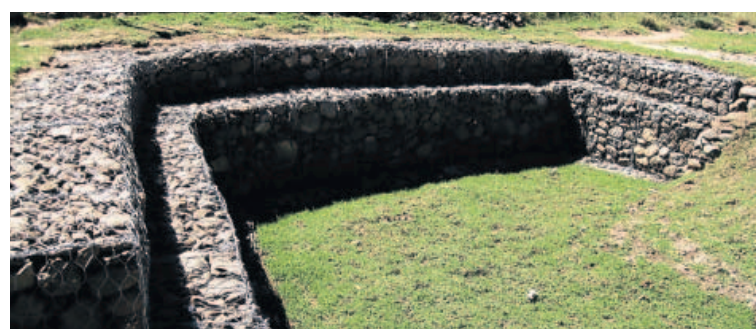
There is an urgent need to rehabilitate, conserve and restore degraded landscapes through sustainable land management.
