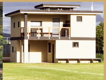
Above: The Knysna Light House is fire-proof, bullet-proof, superior strength, better acoustic and thermal properties, termite-resistant, made primarily (75%) from chipped invasive biomass by the Value-Added Industries programme.
