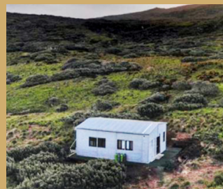
Above: The Gough Island Emergency Hut is made from wood-plastic composite, with finishings using invasive wood, by the Value-Added Industries and Eco-Furniture Programmes.
