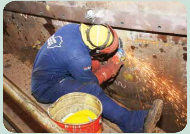
Above: The president visited the South African shipyards during his Operation Phakisa tour and witnessed the super tugboats that are being built there.
