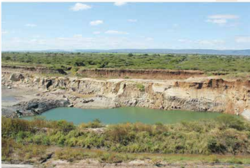
Picture 4: Unlawful commencement of an EIA listed activity and unauthorised water uses.
