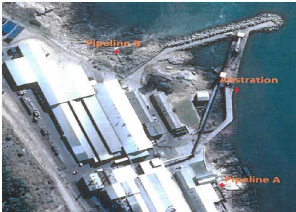
Figure 1: Aerial view of the two discharge points (Pipelines A and B) Before upgrade of the pipelines
