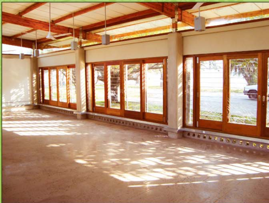
Uncluttered internal space, with North wall made up of sliding doors for natural ventilation
