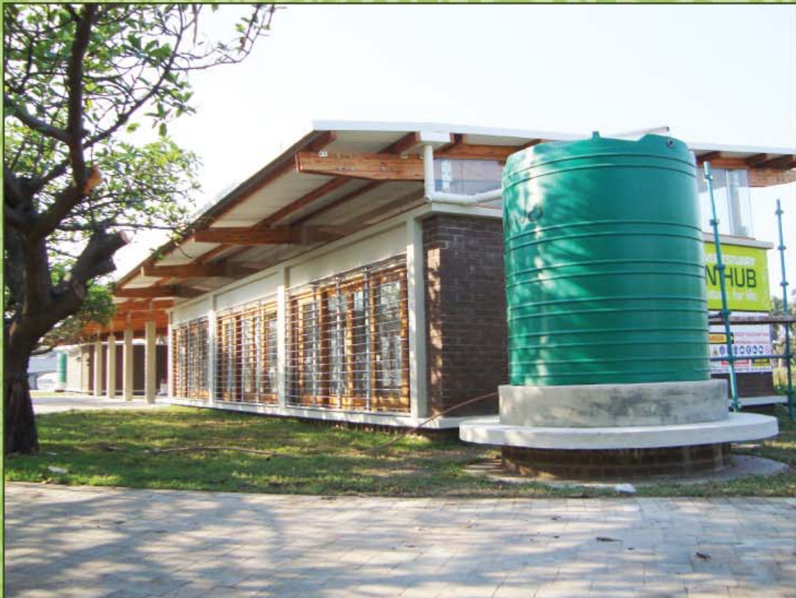
North facing wall of the Green Hub Office showing Rainwater Tank
