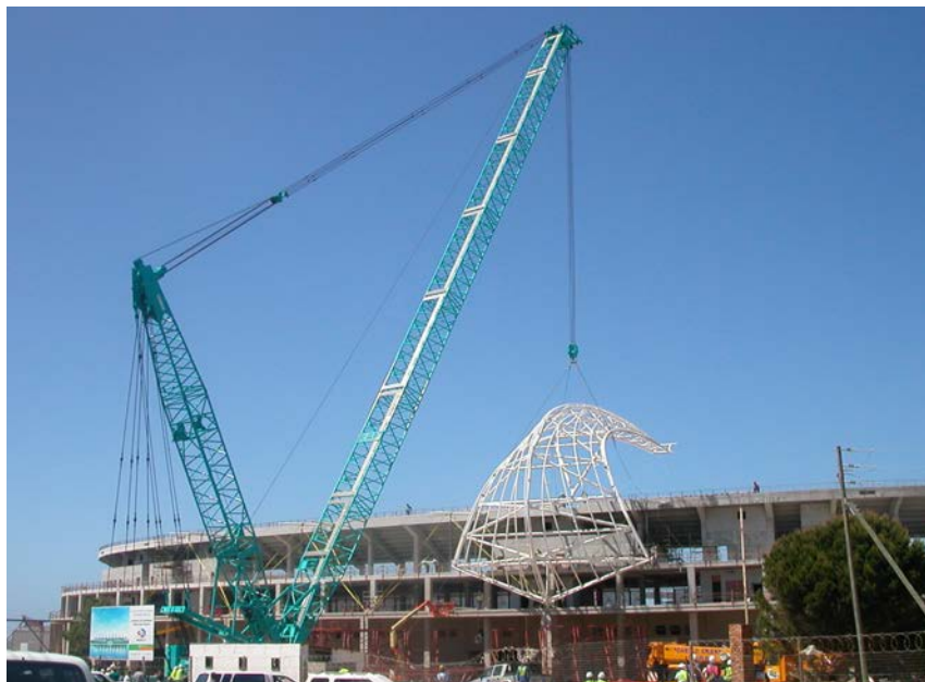
Construction of Nelson Mandela Bay stadium - Port Elizabeth
