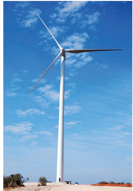
First Electrawinds Wind Turbine at Coega IDZ.
