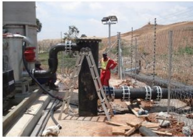
9. Installation of compound Knock-out pot
