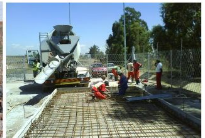
10. Casting of generator slab
