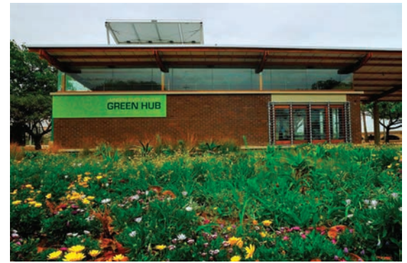
Umgeni River Estuary Green Hub Building (eThekweni Municipality, 2010)
